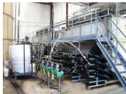
600 GPM Poultry Further Processing Phys/Chem System
